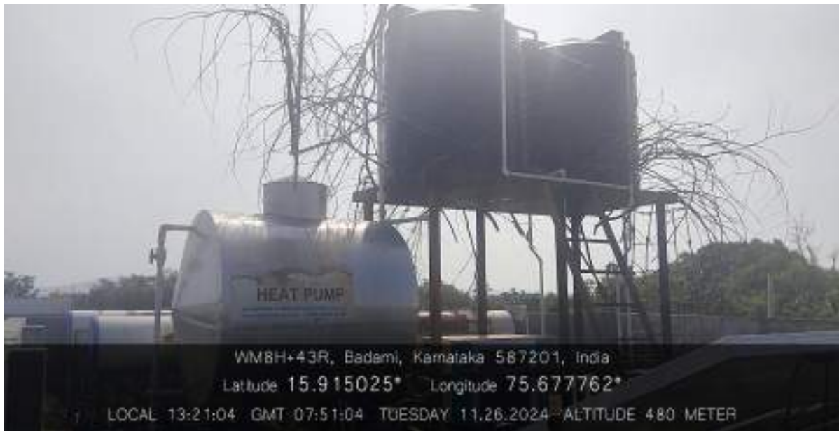
Overhead Syntex tank for supply of hot water
